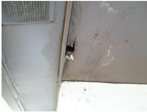
8. Damaged Eave
