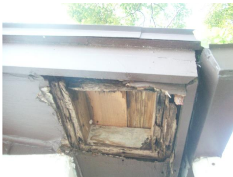
35. Damaged Eave
