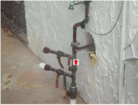
85. Shut Off Leak
