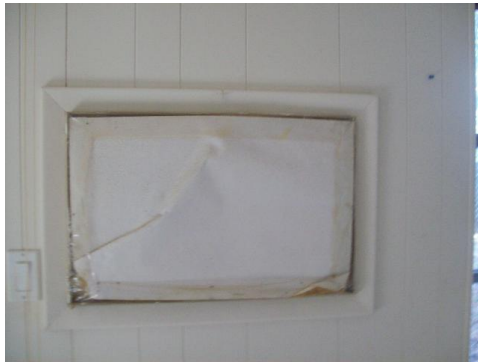
56. Window Unit Covered
