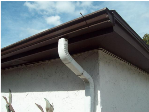
31. Gutter And Downspout
